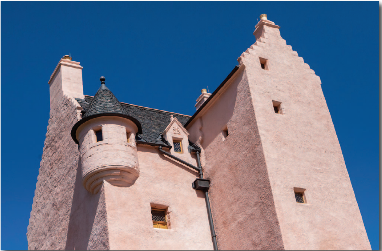
A fine example of the modern stonemasons' skill, blending the old with the new in the restoration of Fairburn Tower.
